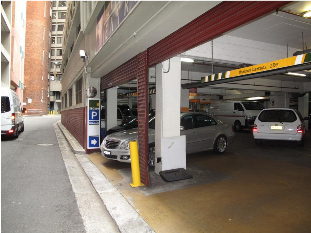
Figure 2.8: Ground level parking at 33-35 Pitt Street, off Underwood Street. C&L 2011.
